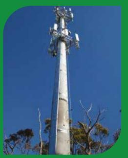
ICP produces spun prestressed concrete poles which are used by communication companies to distribute the signal through cable to their customers. place where there is a risk of cable movement in high wind conditions. Engineered concrete communication poles from ICP are light-weight, noncombustible, termite proof and corrosion proof which are ideal for Tanzanian environments
